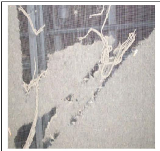
Cottonwood Seed & Other Debris Simply rolls off of Air Intake Filters
