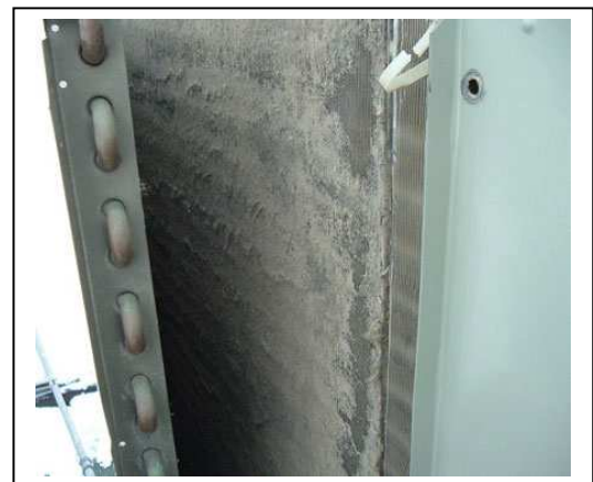
Split Coil System with a Dirty Inner Coil
