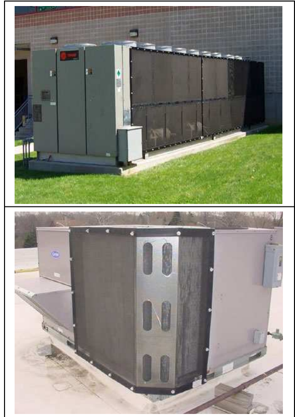
Air Cooled Chiller & Condenser units shown with coil filters that isolate debris on the outside of unit for quick & easy cleaning. Coils stay clean all season long.
